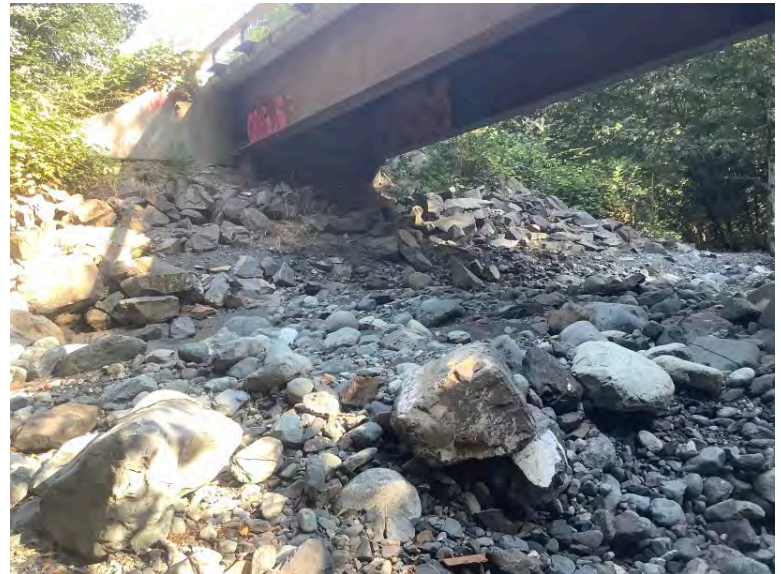
Left Bank Abutment when facing downstream
