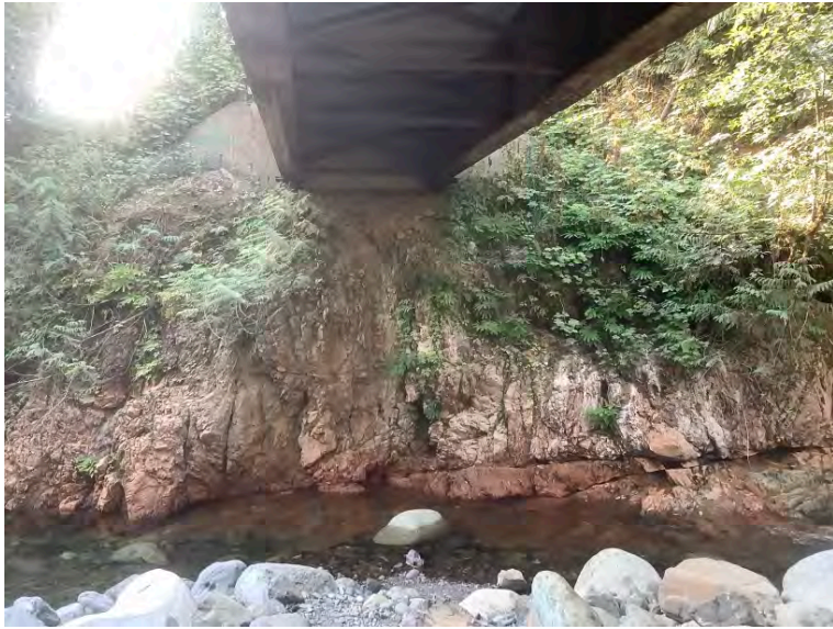
Right Bank Abutment when facing downstream
